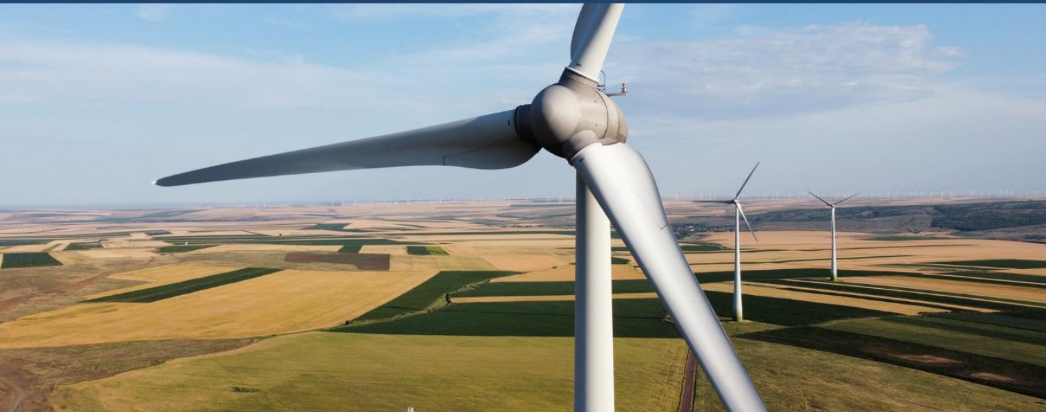
Premier Energy's 80 MW Wind Park, Mihai Viteaz, Constanta County, Romania
